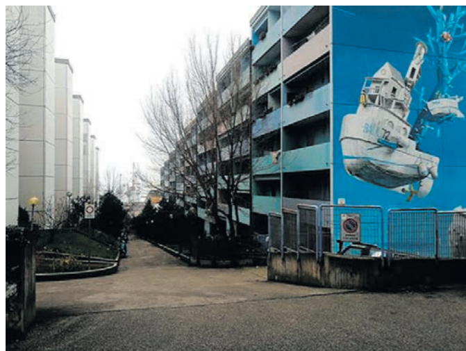
Ponziana ATER complex, installation of 183 photovoltaic panels.
