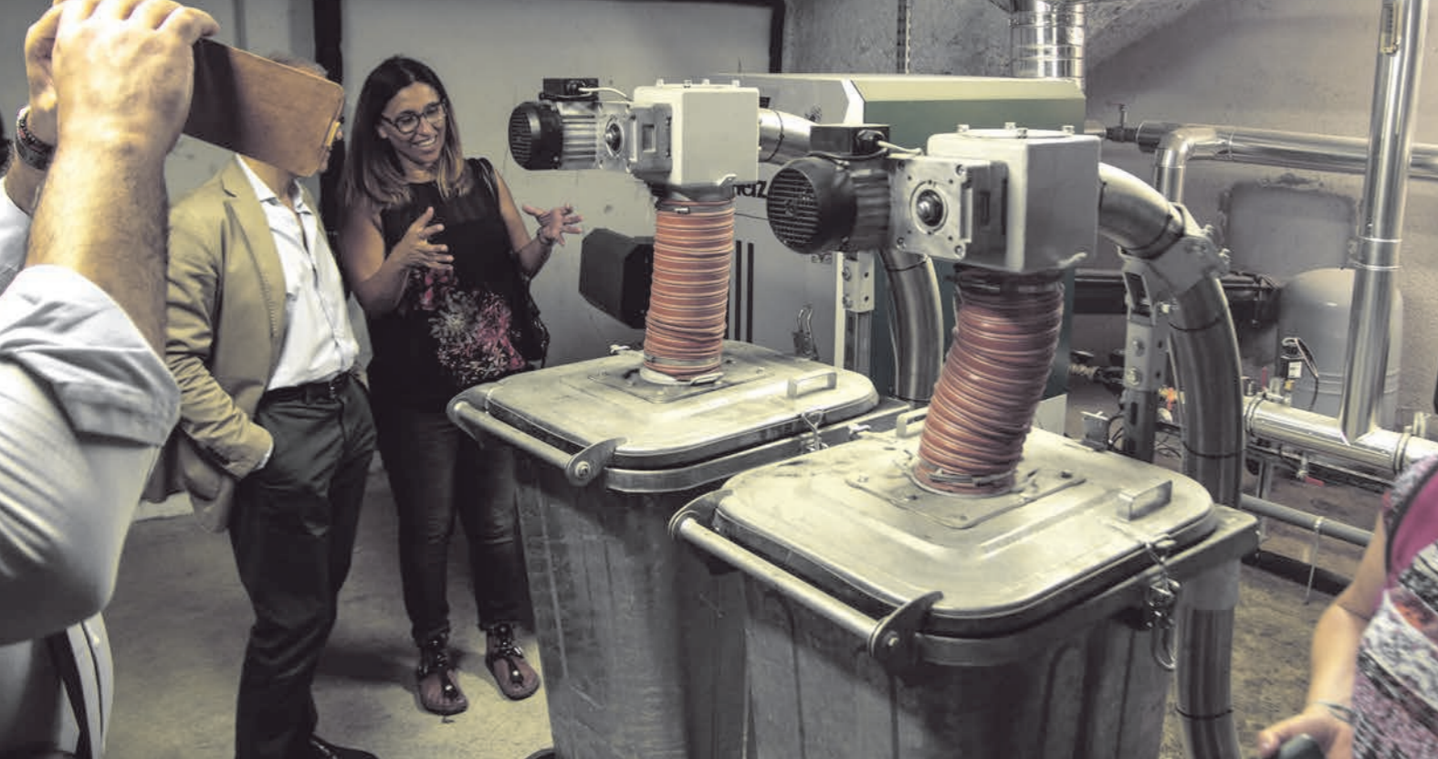
Claudia Mazzoli, project manager for the Emilia-Romagna Region, Italian partner of the SHERPA project, shows the good practices of energy efficiency in public buildings developed in her region.
