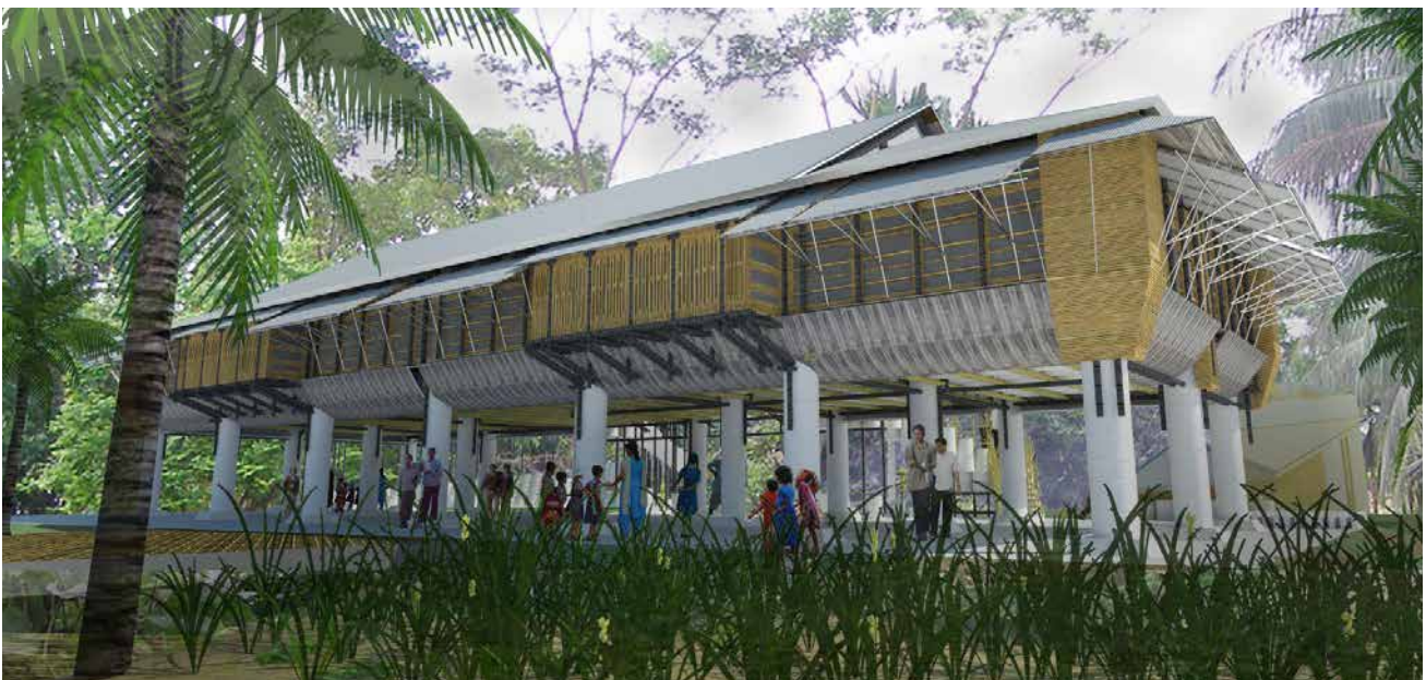
FIGURE 39. Shelter of kindness – Proposed multipurpose hall in Bangladesh which also functions as a raised emergency shelter. The building would rest on pillars and has buoyant tanks that raise it up during floods. (Image: GiantGrass, 2011, permission granted - https://www.giantgrass.com/project/shelter-of-kindness-2/ )
