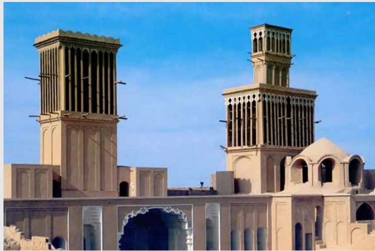
FIGURE 23. Central wind tower with water for cooling for use in hot and dry climates (Image from Kamal, 2012) 127
