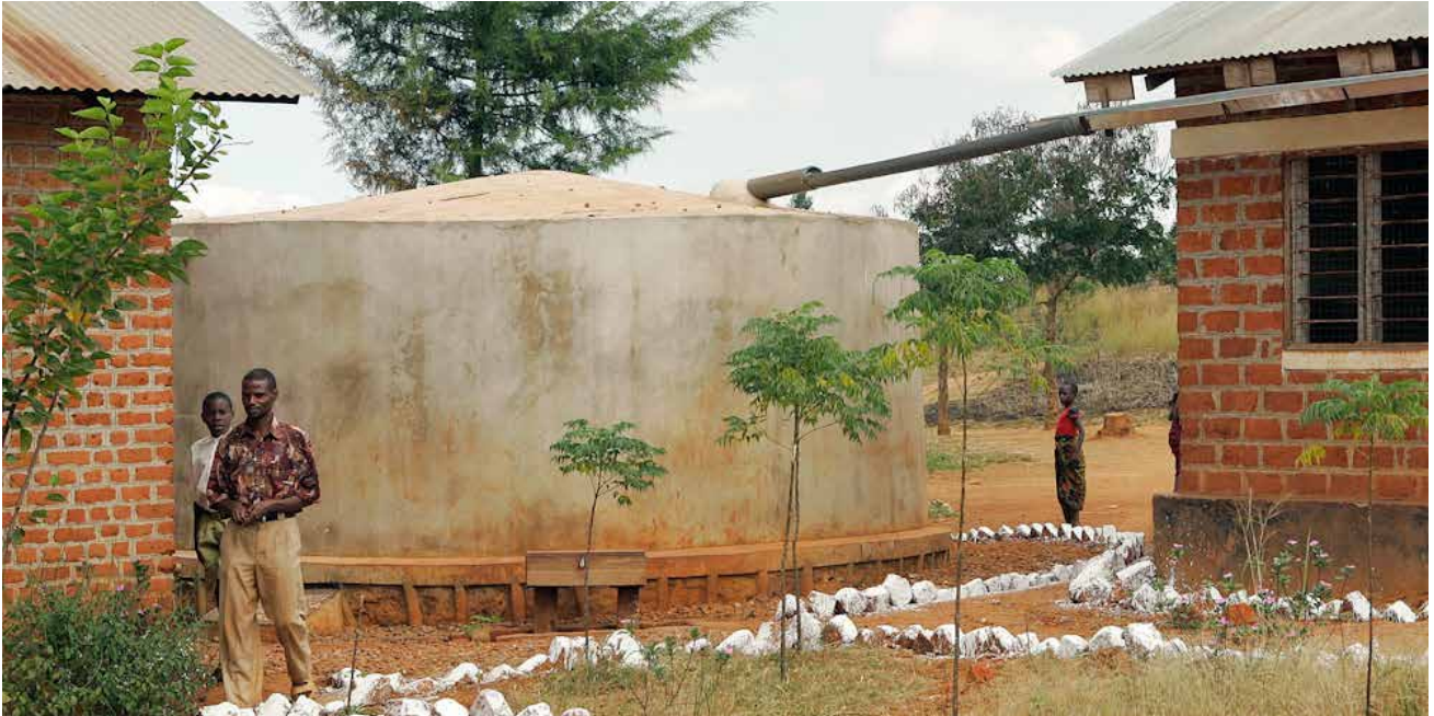
FIGURE 34. Rainwater harvesting tank, Uganda (Image from: Baguma et al., 2012) 148
